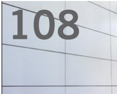
Internal Wall Covering RAM 2011-2014
